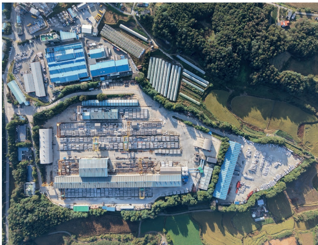
Aerial view of Daewoo ST production site in Jincheon, South Korea
