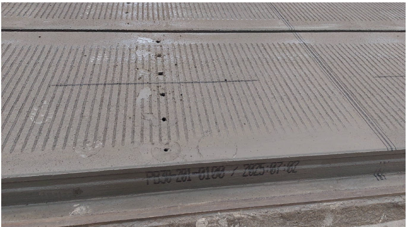
Hollow core slabs with marks and weep holes immediately after element casting
