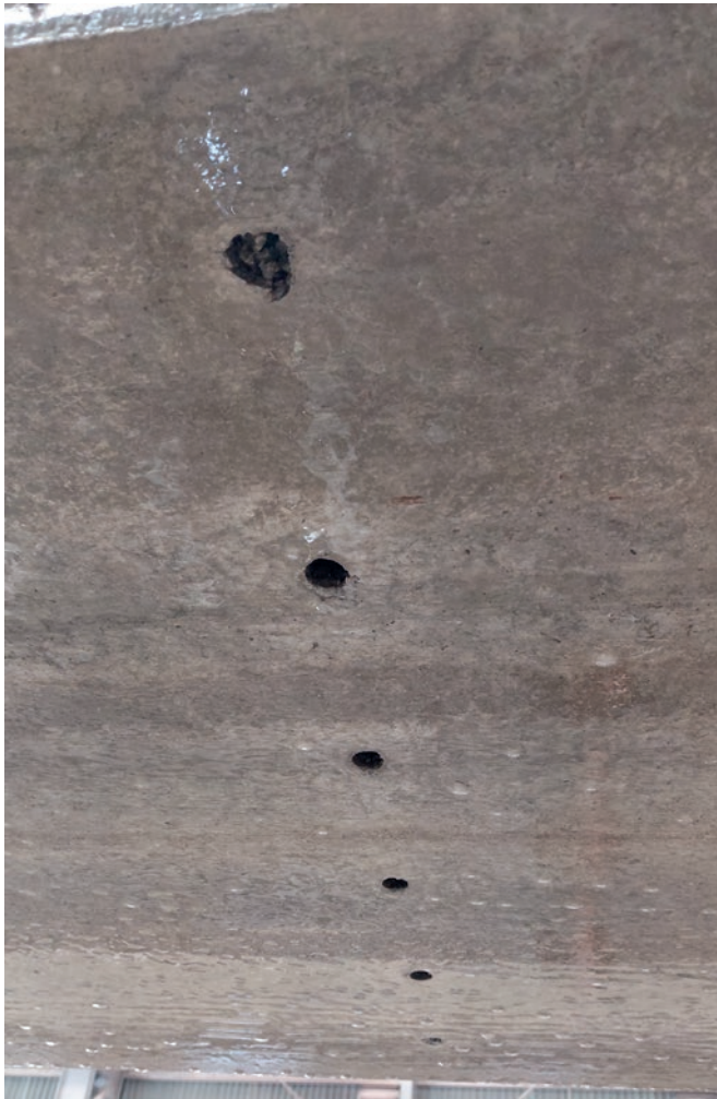
Weep holes as seen at the underside of the hollow core slabs
