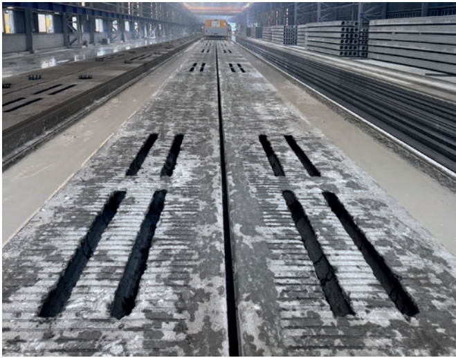
Daewoo ST production hall with four long casting beds
